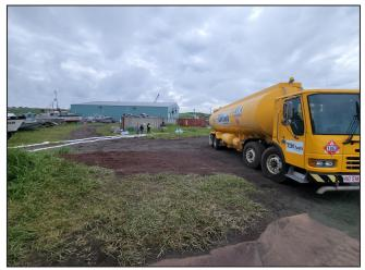
**Photo 3:** Sorbent boom placed to assist with berming until trenches are dug.
