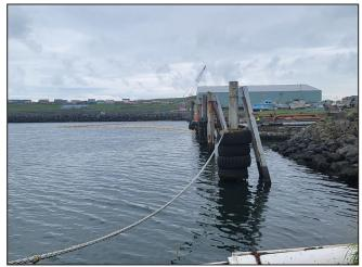
**Photo 8:** The containment boom is in place and anchored.
